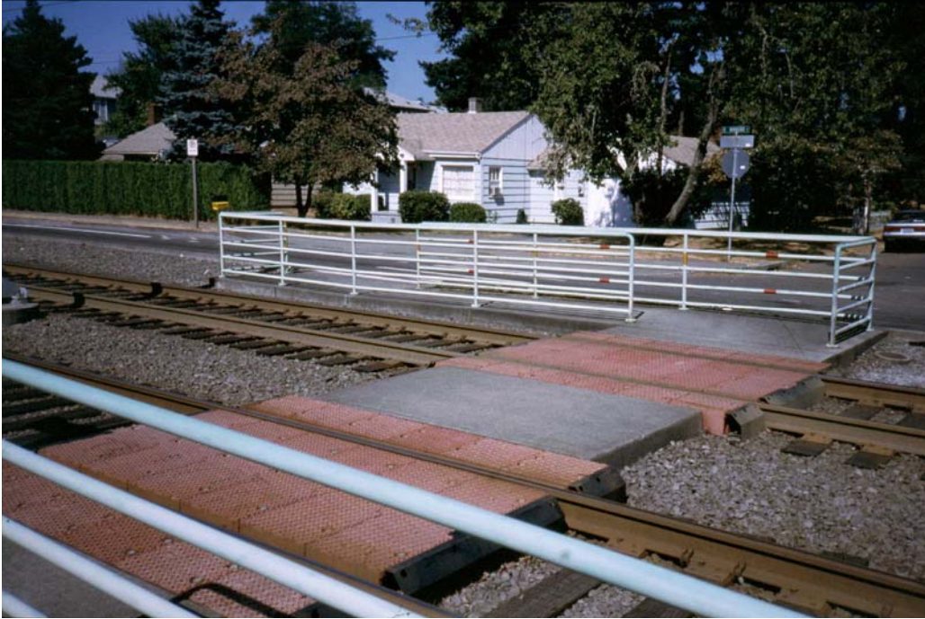
Houston: Pedestrian Z-Crossing Under Construction
